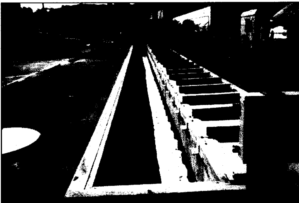
Figure 2-4 Escondido MS Delaware Sand Filter
